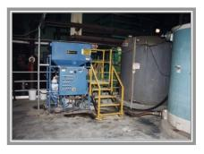
The next step in the dewatering process is to squeeze the water out of the sludge with diaphragm filter presses. The
