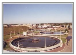
The secondary treatment facilities are comprised of Oxygenation Tanks, Pure Oxygen Generating Plant, Liquid Oxygen Storage Tanks, Secondary Clarifiers, Return Sludge Pumping Station and Splitter Box, Sludge Thickeners, Pumping Station, Sludge and the Dewatering Building Addition.
